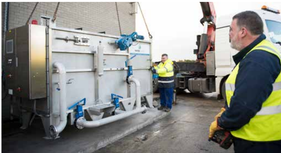
Picture shows our 5m 3 /h DAF being lowered into position
